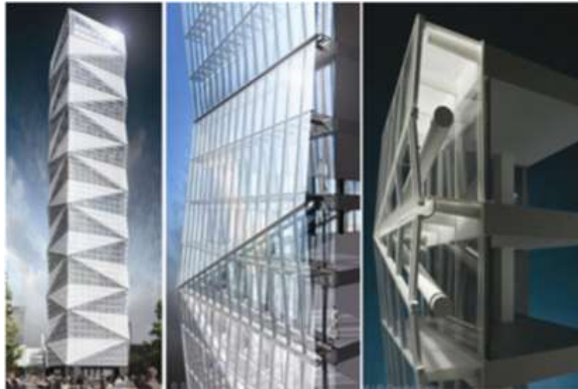
Figure 3: Jinao Tower in Nanjing, China (Courtesy of Skidmore, Owings & Merrill LLP)
